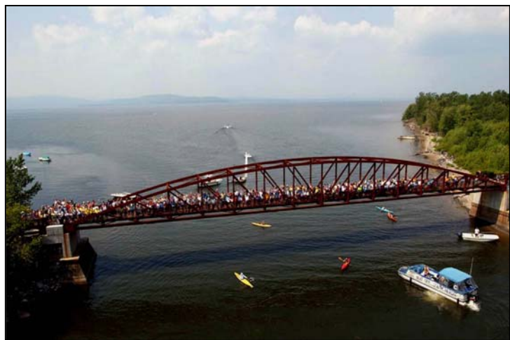
Burlington & Colchester Trail Bridge Photo: Local Motion
