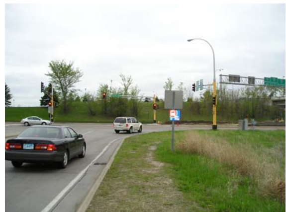
Bus Stop with no Pedestrian Facilities – Roseville
