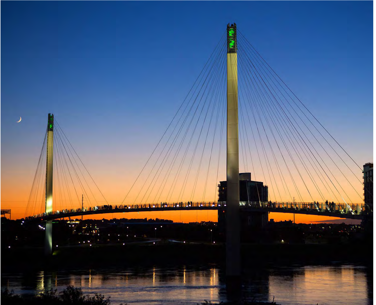
Bob Kerrey Pedestrian Bridge connecting Iowa and Nebraska | Photo by Matthew Nissen
