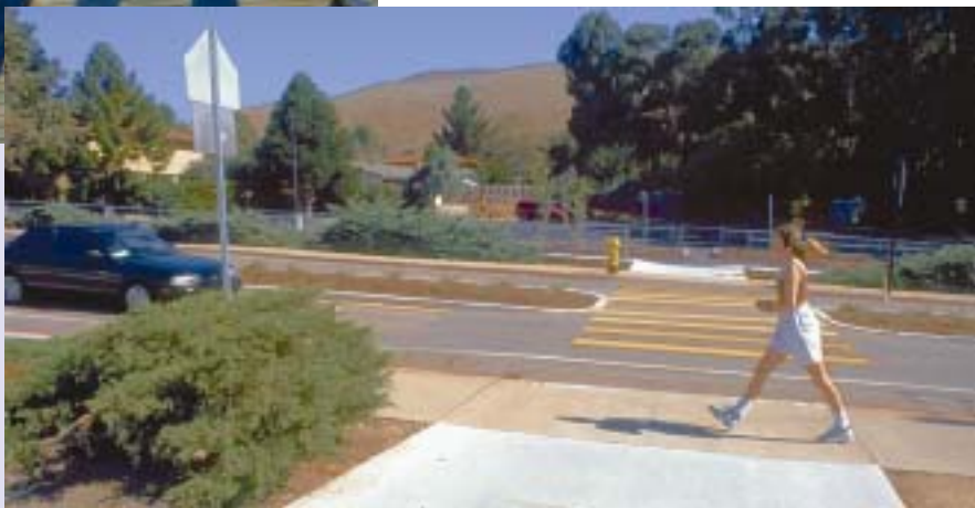
Crosswalk on speed table with median
