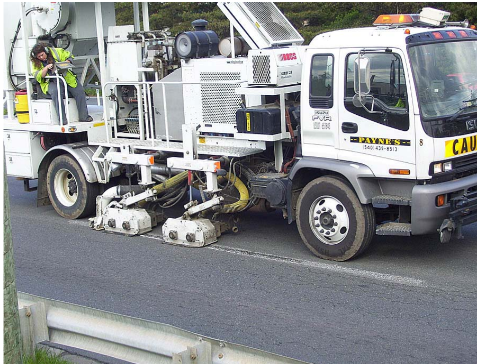
Figure D-3. Eradication of Skip-Lines on Sterling Boulevard
