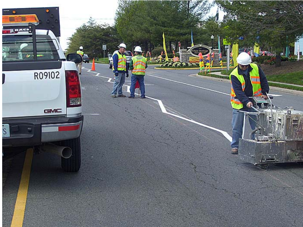
Figure D-6. Marking Painting on Westbound Approach of Sterling Boulevard
