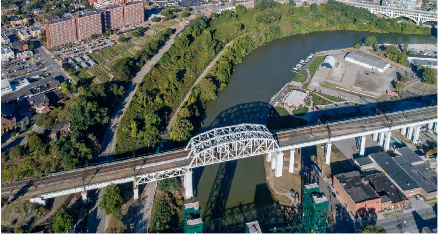
An aerial view of Irishtown Bend before hill stabilization | Photo courtesy LAND Studio
