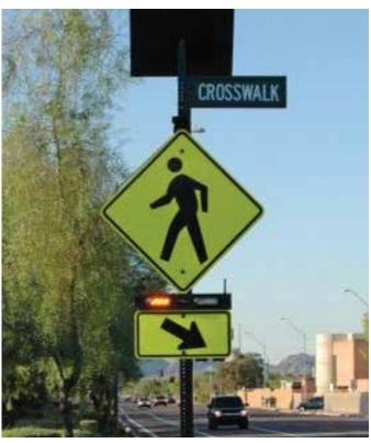
An example of a flashing beacon to alert drivers of the presence of crossing pedestrians | Photo courtesy Institute of Transportation Engineers
