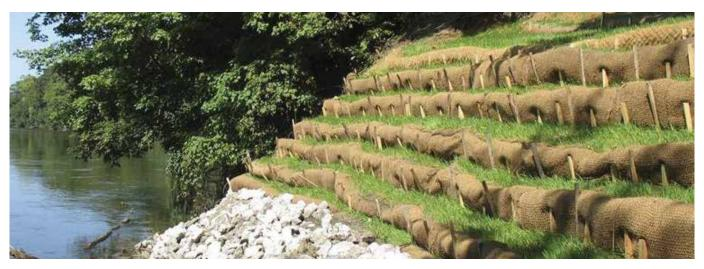
An example of terracing and slope stabilization | Photo courtesy NBAC
