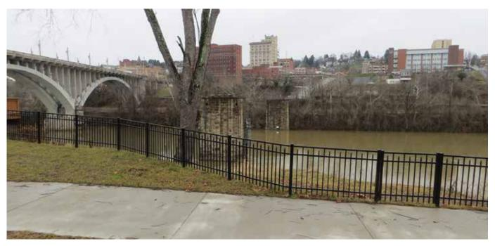
The Nickel Bridge (or Low Level Bridge) in Fairmont, West Virginia, was removed, but a new bridge can be constructed on the remaining abutments. | Photo courtesy RTC
