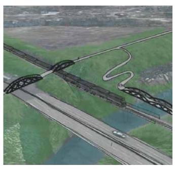
A rendering of Option 2, including all three new bridges needed to cross US 50, the active CSX line and the West Fork River | Photo courtesy NBAC
