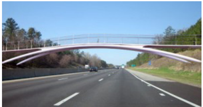
The ATT bridge over I-40 is only the second arch-support, stress-ribbon bridge in the US. (Photo courtesy East Coast Greenway)
