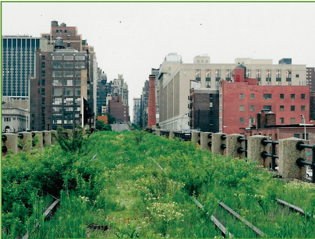
High Line - a railbanked corridor in New York City
