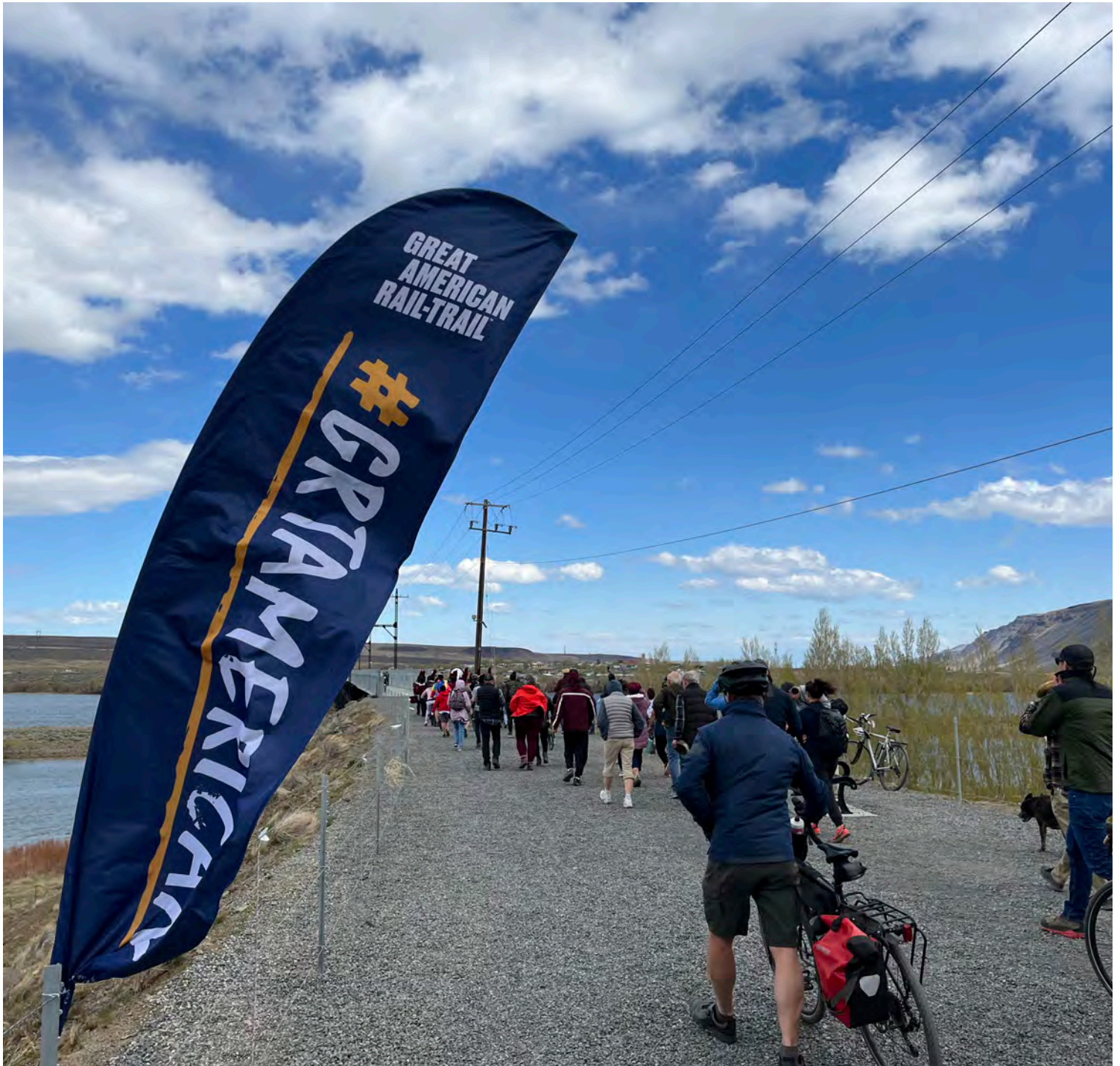
The Beverly Bridge opened for trail use across the Columbia River along the Palouse to Cascades State Park Trail in April 2022. | Photo by Kevin Belanger
