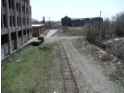
Jefferson Avenue E., southeast view.
