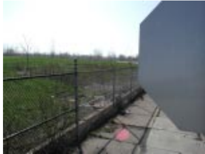
Terminus at Jefferson Avenue E., southeast view.
