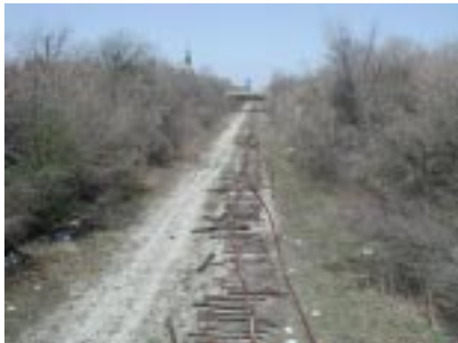
Pedestrian bridge from Lafayette Street, northwest view.
