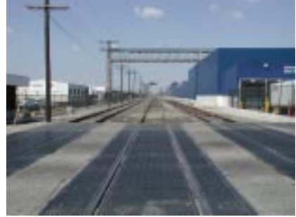
Holbrook Avenue, northwest view.
