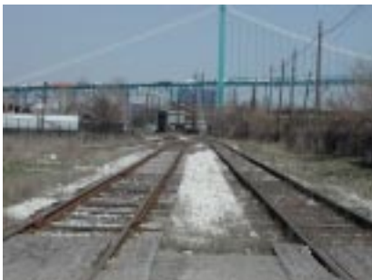
Scotten Street, northeast view.
