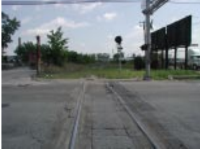
Oakland Avenue, northeast view.
