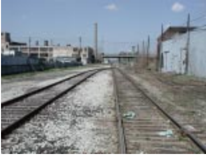
Trombly Street, northwest view.
