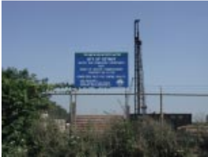
Freud Street and Clairpoint Street, southeast view.
