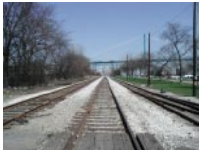
Jefferson Avenue W. and Grand Boulevard W., northeast view.
