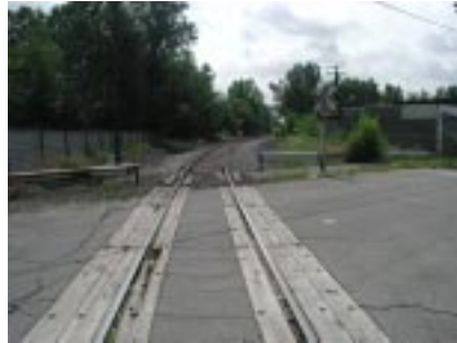
Dwyer Street and Brimson Street, southeast view.
