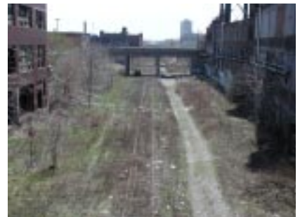
Wilkins Street, southeast view.
