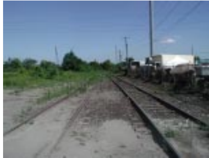
Freud Street and Clairpoint Street, southeast view.
