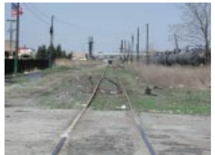
Ferry Street E., northwest view.
