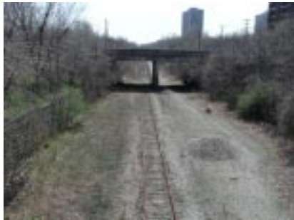
Antietam Street, southeast view.
