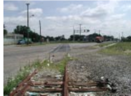
Main Street and McNichols Road, northeast view.
