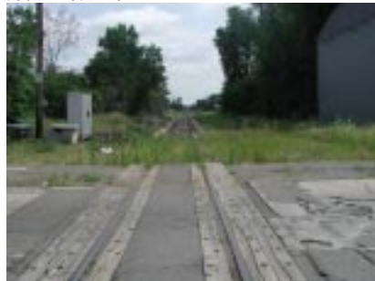
Goddard Street south of McNichols Road, northeast view.
