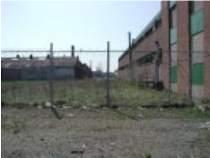
Warren Avenue E. between Bellevue and Beaufait Streets, southeast view.
