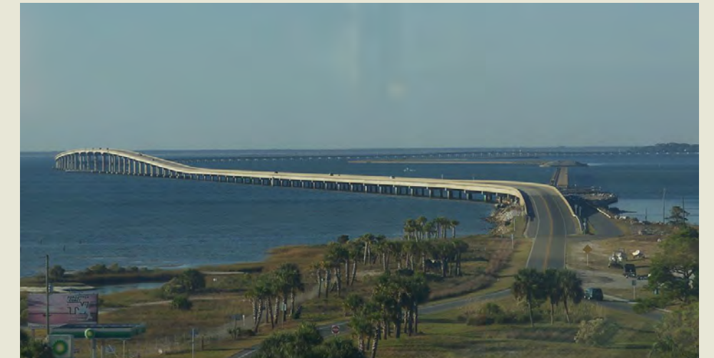
The St. George Island Bridge spanning Florida’s Apalachicola Bay provides another example of enabling active transportation through bridge design. The 4.1 mile long bridge opened in 2004 includes 10 foot shoulders accessible to bicyclists. Source: By Ebyabe - Own work, CC BY-SA 3.0, https://commons.wikimedia.org/w/index.php?curid=12133923
