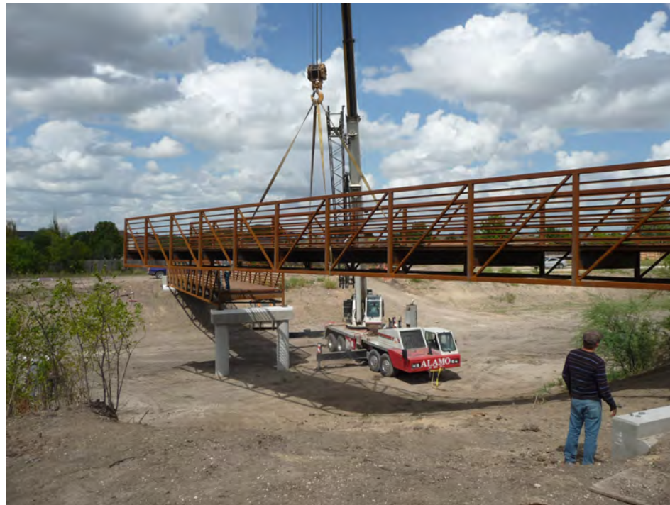
Pre-fabricated bicycle and pedestrian bridges generally span distances of between 50 and 200 feet Photo by Halff Associates
