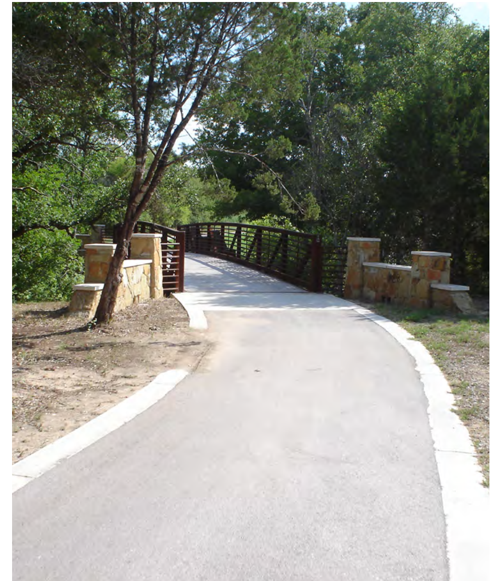
Each segment of the proposed LRGV regional active transportation network will be built according to varying design criteria based on location, surrounding conditions, user type, and cost. Photo by Halff Associates
