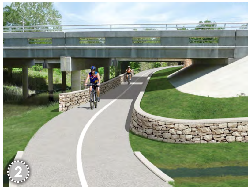
The placement of multi-use trail underpasses along drainage ditches is increasingly common (picture 1). Retrofitting existing underpasses may require substantial grading and embankment stabilization (picture 2). The proposed Arroyo-Resaca Multi-use Trail Segment (page 3-38) would have to pass under FM1846 to connect San Benito and the Arroyo Colorado (picture 3). Source: Halff Associates
