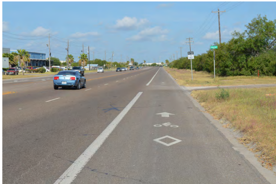
Some shoulders on TxDOT highways in Cameron County have been converted to designated bicycle lanes. Photo by Halff Associates
