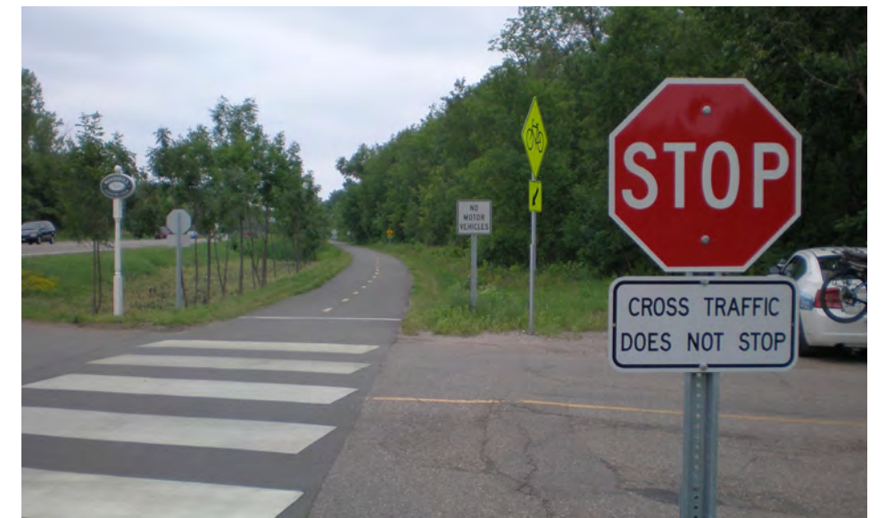
Mid-block bicycle and pedestrian crossings in urban environments (top right) may warrant the use of pedestrian-activated signals or flashing beacons. Trail crossings in rural locations may simply require the installation of pavement markings and signage (bottom right), particularly where low traffic volumes are expected. Photos by Halff Associates (top); Danny McCullough (bottom)
