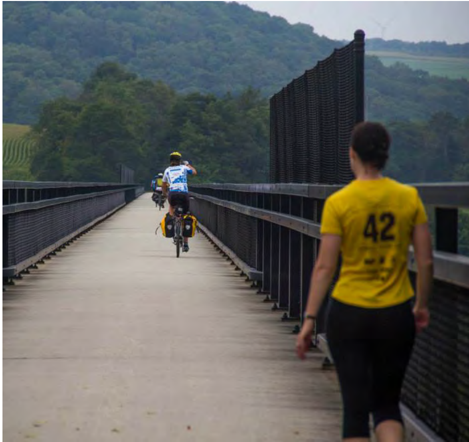
One of the many highlights along the Great Allegheny Passage is this high trestle bridge. Photo by Saara Snow
