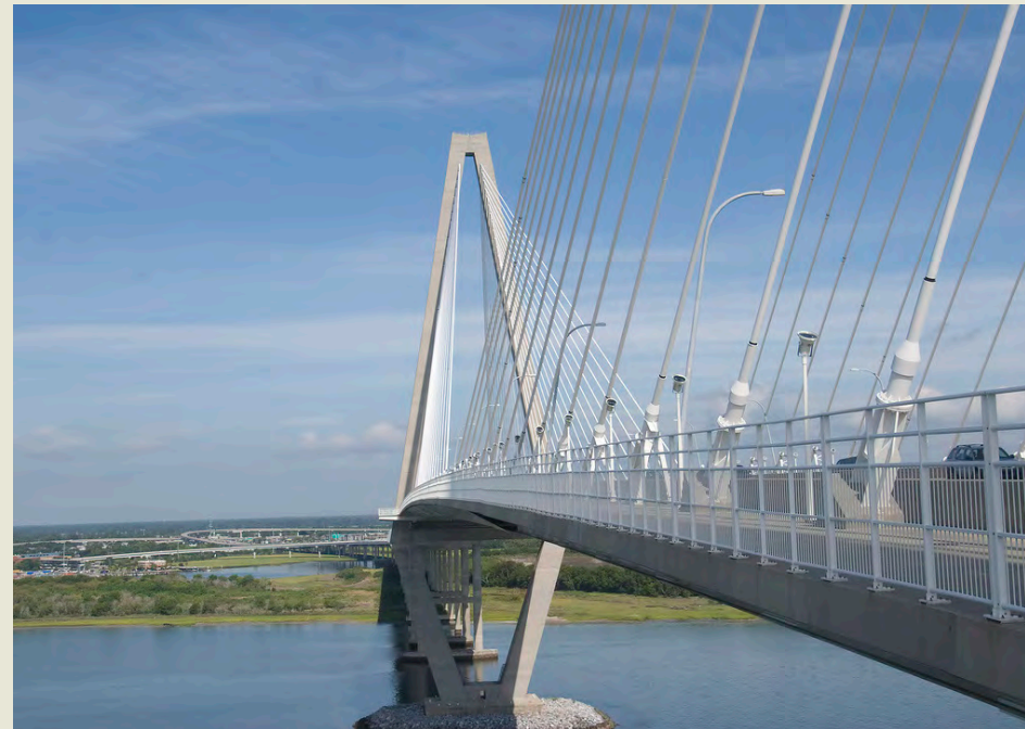
South Carolina’s Arthur Ravenel Jr. Bridge includes viewing decks and a two-way bicycle and pedestrian path (sometimes referred to as the “Wonders’ Way.”) Source: Flickr: Arthur Ravenel Jr. Bridge Charleston (SC), Ron Cogswell, 2012
