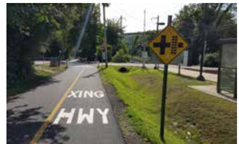
Pavement marking improvements to trail intersections near Spring Mill in Whitemarsh Township.
