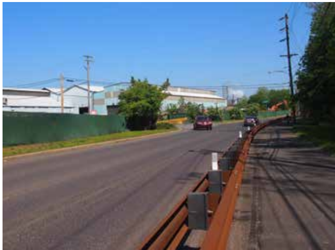
Photo 19: View of the guardrail barrier along the eastern trail segment at the intersection of Keim Street and Industrial Highway.
