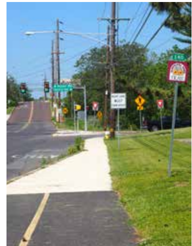
Photo 20: View of the eastern segment of trail looking north towards the intersection of Moser Road and Industrial Highway.
