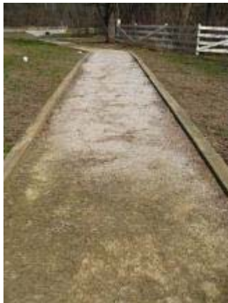
Photo 38 Soiltac Powder Mix-In almost two years after installation. March 17, 2009.
