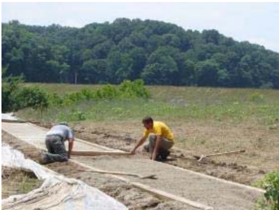
Photo 59 Soiltac Liquid Mix-In trail segment is leveled. June 27, 2007.
