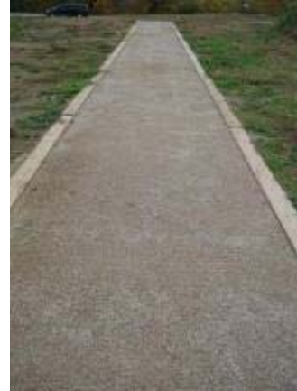
Photo 140 Three Quarter Inch Minus Base and Quarter Inch Minus Top Limestone trail segment maintained itself in dry temperatures. October 19, 2007.
