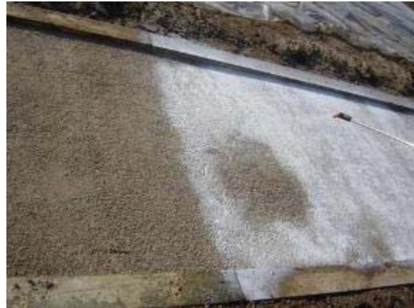
Photo 44 Soiltac Liquid Topical has a penetration depth of 1/8 inch. June 27, 2007.
