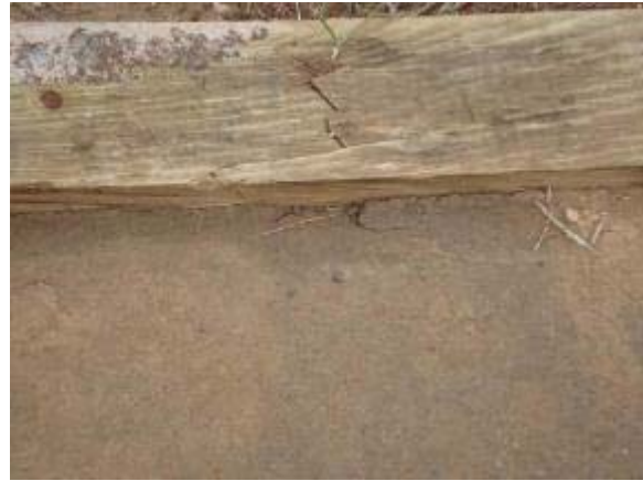
Photo 97 StaLok trail segment maintained itself through first round of testing. October 19, 2007.
