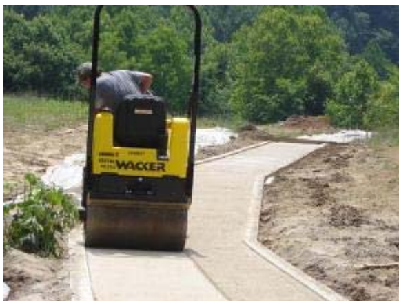
Photo 32 Soiltac Powder Mix-In is smoothed and compacted. June 27, 2007.
