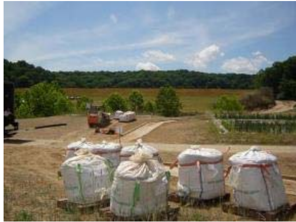
Photo 70 Stabilizer arrives pre-mixed with ¼ inch minus aggregate. June 19, 2007.
