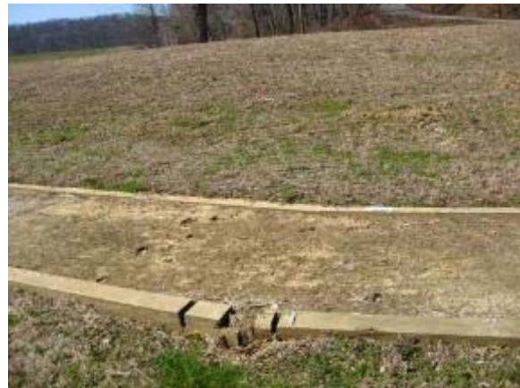
Photo 39 Soiltac Powder Mix-In does not have a constructed drainage mechanism considered appropriate for trail construction. March 17, 2009.
