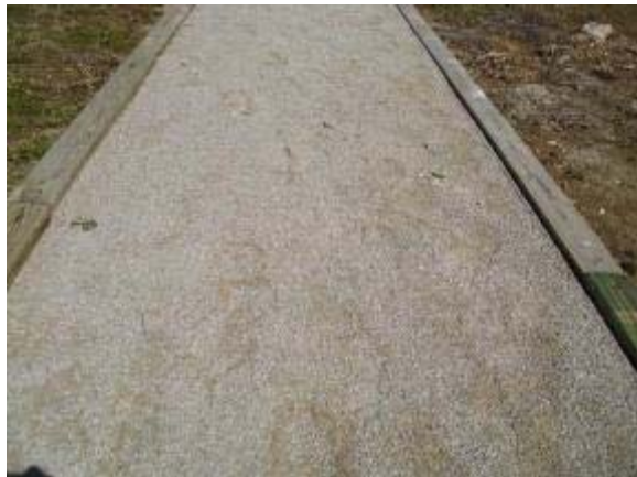
Photo 141 Three Quarter Inch Minus Base and Quarter Inch Minus Top Limestone trail segment after heavy rain. March 13, 2008.
