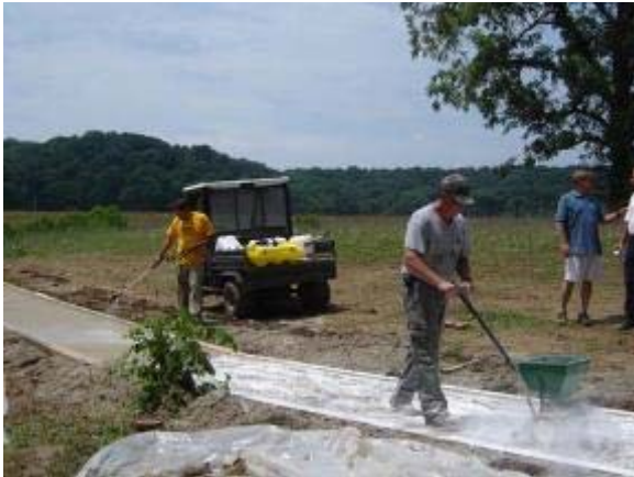
Photo 55 Soiltac Liquid Mix-In is applied to a base of 2 inches of native soil. June 27, 2007.
