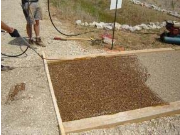
Photo 7 Top dress is sprayed with Klingstone 400 to seal the pea gravel. June 16, 2007.
