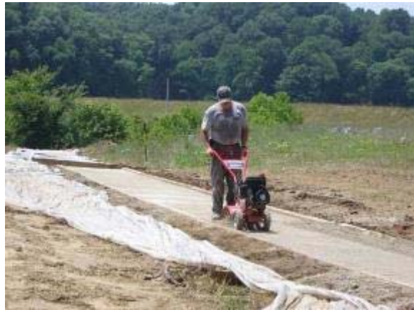
Photo 58 Soiltac Liquid Mix-In surface is tilled. June 27, 2007.
