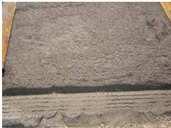
Photo 74 Stabilizer trail segment is prepared. June 21, 2007.
