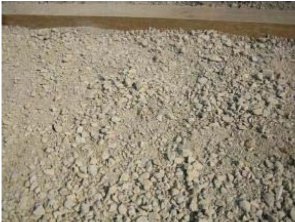
Photo 122 Three Quarter Inch Minus Limestone trail segment is composed of two three inch lifts with 50 percent dust. August 1, 2007.
