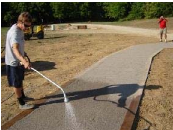
Photo 73 Stabilizer trail segment is prepared. June 21, 2007.
