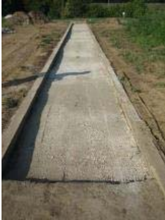
Photo 139 Three Quarter Inch Minus Base and Quarter Inch Minus Top Limestone trail segment is composed of 4 inch base; and a 2 inch top-dressing. August 9, 2007.
