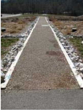
Photo 13 Klingstone almost two years after installation has small amount of loose fines coming to surface. March 17, 2009.
