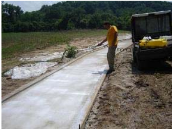
Photo 34 Soiltac Powder Mix-In is sprayed to seal the surface. June 27, 2007.
