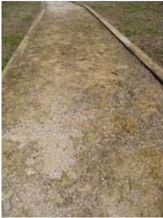
Photo 26 Soiltac Powder Topical almost two years after installation. March 17, 2009.
