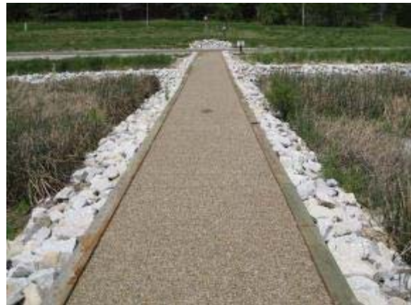
Photo 12 Klingstone surface almost a year after installation. May 6, 2008.
