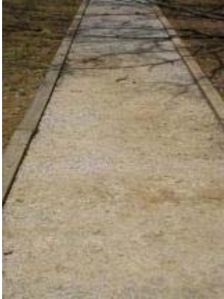
Photo 128 Three Quarter Inch Minus Limestone trail segment where water pooled after rain. March 13, 2008.
