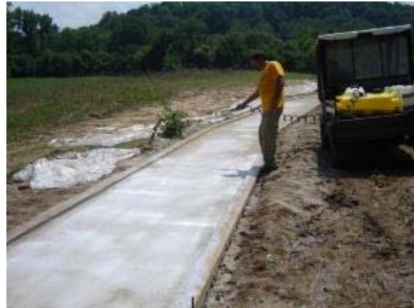
Photo 62 Soiltac Liquid Mix-In trail segment is sprayed to seal with a penetration of 4 inches. June 27, 2007.
