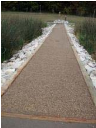
Photo 11 Klingstone amber color has started to fade. October 19, 2007.
