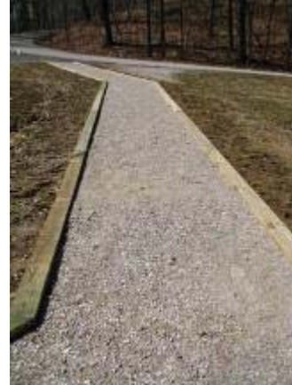
Photo 129 Three Quarter Inch Minus Limestone trail segment where water pooled after rain. March 13, 2008.
