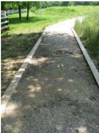
Photo 130 Three Quarter Inch Minus Limestone trail segment almost one year after installation. June 12, 2008.
