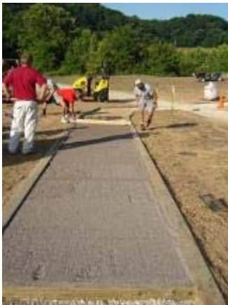
Photo 71 Stabilizer is applied at a 3 inch depth on top of the base. June 21, 2007.
