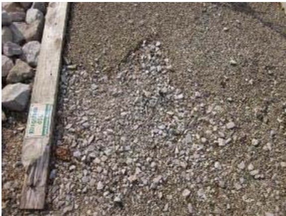
Photo 15 Klingstone at beginning of trail segment has started to wash out. November 22, 2011.
