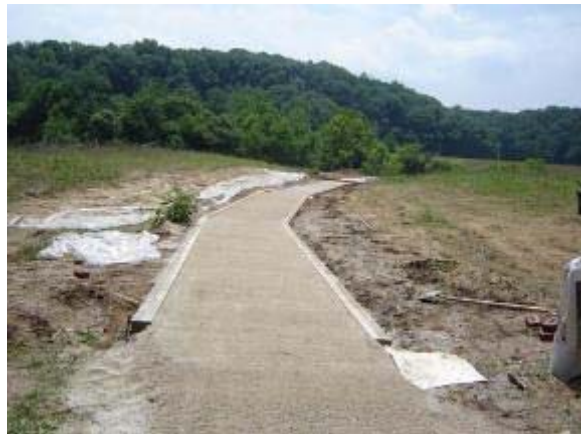
Photo 60 Soiltac Liquid Mix-In trail segment is prepared. June 27, 2007.
