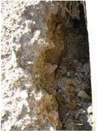
Photo 145 Three Quarter Inch Minus Base and Quarter Inch Minus Top Limestone trail segment after heavy rain. March 17, 2009.
