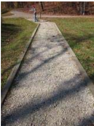
Photo 132 Three Quarter Inch Minus Limestone trail segment showed prevalence of larger fines working their way to the surface. November 2, 2011.
