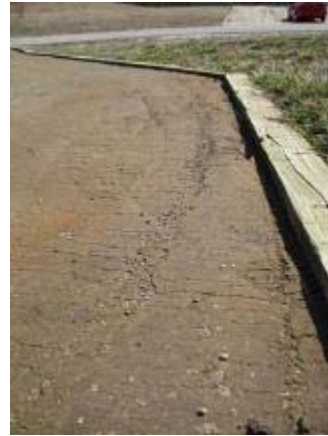
Photo 103 StaLok trail segment previously shown with marks had repaired itself. March 17, 2009.
