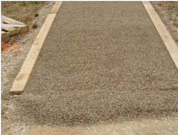
Photo 3 Klingstone top dress preparation of ¾ inch washed pea gravel (round river rock). June 16, 2007.
