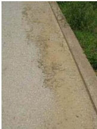
Photo 65 Soiltac Liquid Mix-In more than one year after installation seemed to maintain itself. June 12, 2008.
