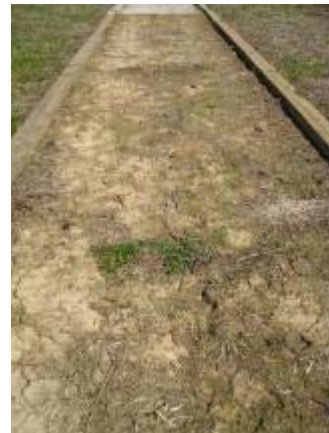
Photo 119 Polypavement trail segment almost two years after installation shows top layer of stabilizer and remaining surface returned to its natural soil base. March 17, 2009.
