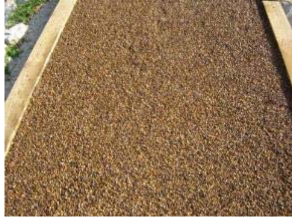
Photo 8 Klingstone 400 has been sprayed to top surface. June 16, 2007.
