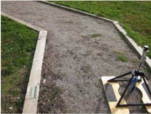
Photo 87 Stabilizer trail segment shows deterioration. November 2, 2011.
