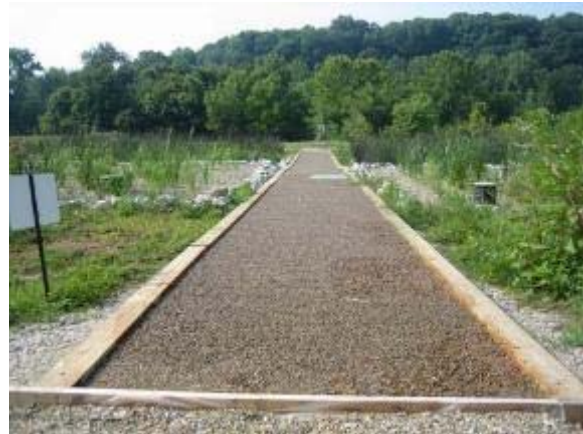
Photo 10 Klingstone trail surface more than a month after installation. August 1, 2007.
