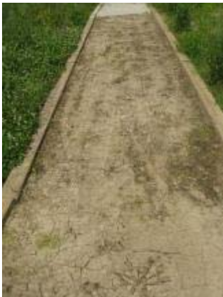
Photo 118 Polypavement trail segment a year after installation shows top layer is all that is left of the stabilizer. June 12, 2008.
