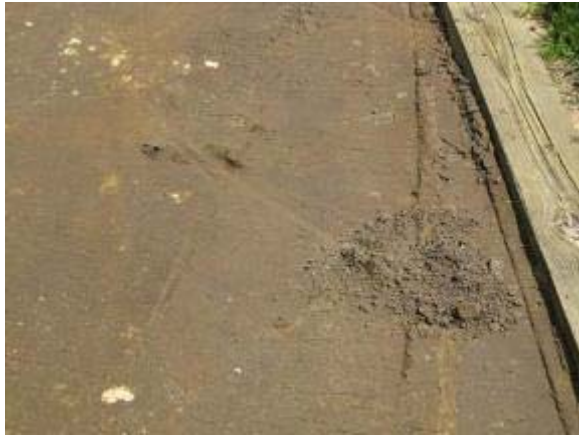
Photo 102 StaLok trail segment with wheelchair marks would repair itself. June 12, 2008.
