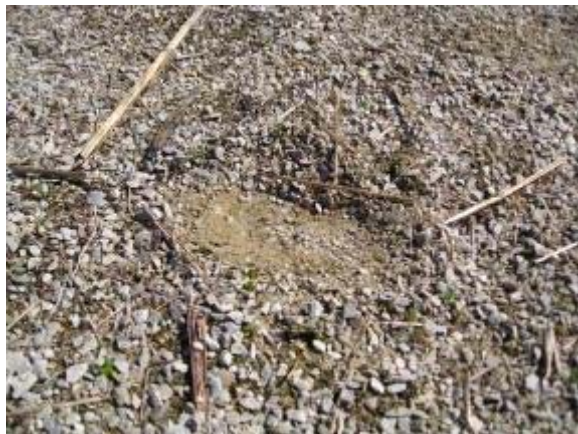
Photo 143 Three Quarter Inch Minus Base and Quarter Inch Minus Top Limestone trail segment showed signs of footprints after heavy rain. March 17, 2009.
