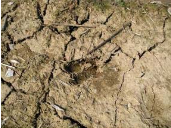
Photo 120 Polypavement trail segment may not have set up properly due to the moist soil of the wetlands. March 17, 2009.
