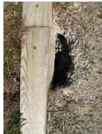
Photo 144 Three Quarter Inch Minus Base and Quarter Inch Minus Top Limestone trail segment after heavy rain. March 17, 2009.
