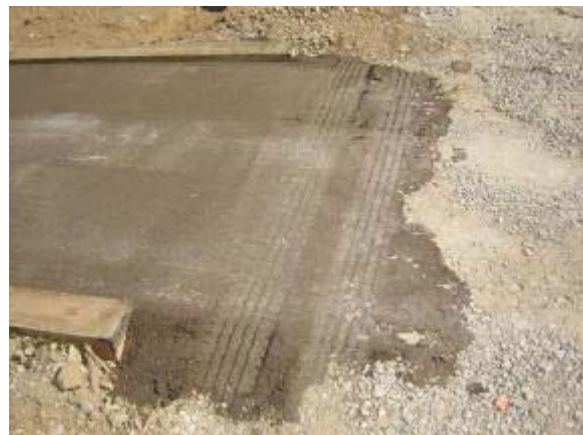
Photo 95 StaLok surface is compacted. June 21, 2007.
