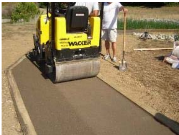
Photo 94 StaLok surface is compacted. June 21, 2007.
