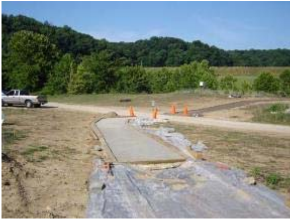
Photo 75 Stabilizer trail segment installation. July 3, 2007.
