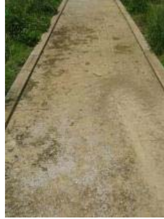
Photo 25 Soiltac Powder Topical one year after installation. June 12, 2008.
