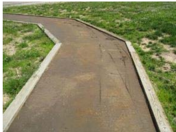
Photo 101 StaLok trail segment with wheelchair marks would repair itself. June 12, 2008.
