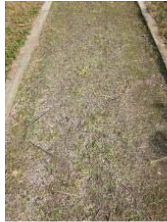
Photo 27 Soiltac Powder Topical more than four years after installation. November 2, 2011.
