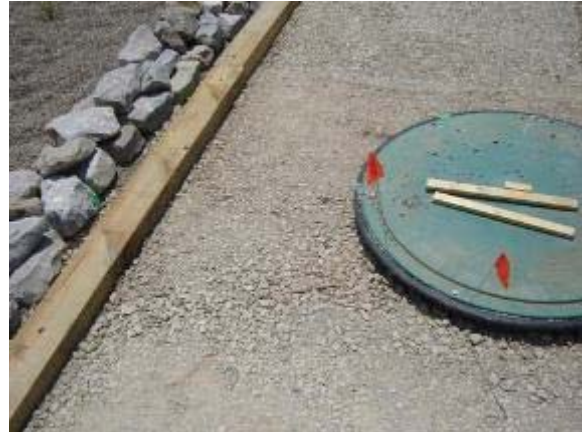
Photo 2 Klingstone base preparation of ¾ inch minus limestone and dust. June 13, 2007.
