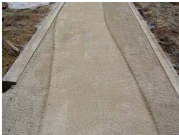
Photo 33 Soiltac Powder Mix-In is smoothed and compacted. June 27, 2007.
