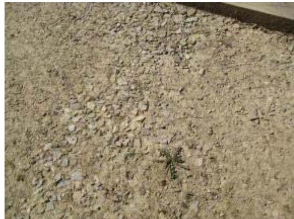
Photo 131 Three Quarter Inch Minus Limestone trail segment remained firm under foot. March 17, 2009.
