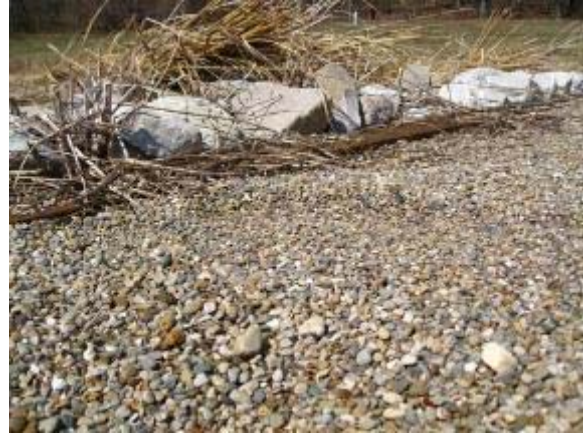
Photo 14 Klingstone loose fines coming to surface. March 17, 2009.
