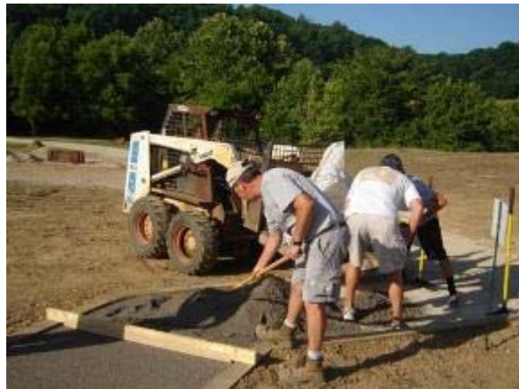
Photo 72 Stabilizer trail segment is leveled at installation. June 21, 2007.
