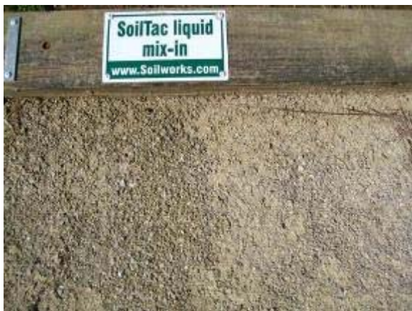
Photo 63 Soiltac Liquid Mix-In trail segment seemed to maintain itself well. March 13, 2008.
