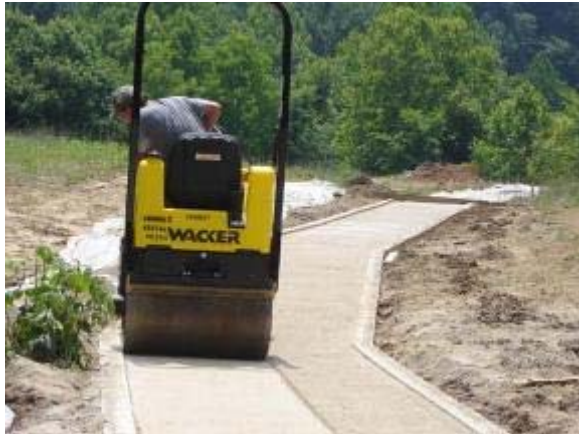
Photo 61 Soiltac Liquid Mix-In trail segment is compacted. June 27, 2007.
