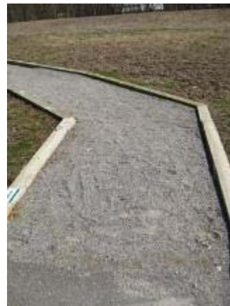
Photo 84 Stabilizer trail segment almost two years after installation. March 17, 2009.
