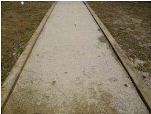
Photo 36 Soiltac Powder Mix-In trail segment maintained its condition a year after installation. March 13, 2008.
