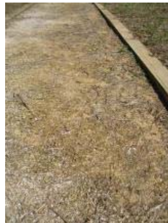
Photo 52 Soiltac Liquid Topical trail segment showed runoff. March 17, 2009.
