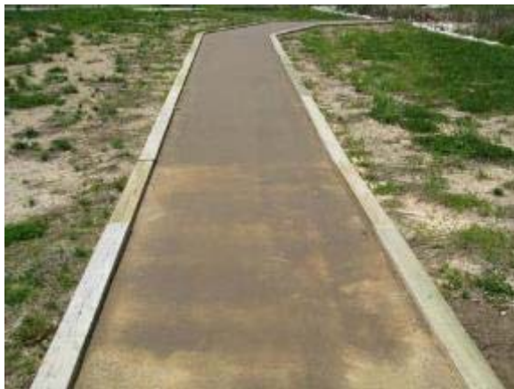
Photo 100 StaLok trail segment was noted for showing indentations and then repairing itself. May 6, 2008.
