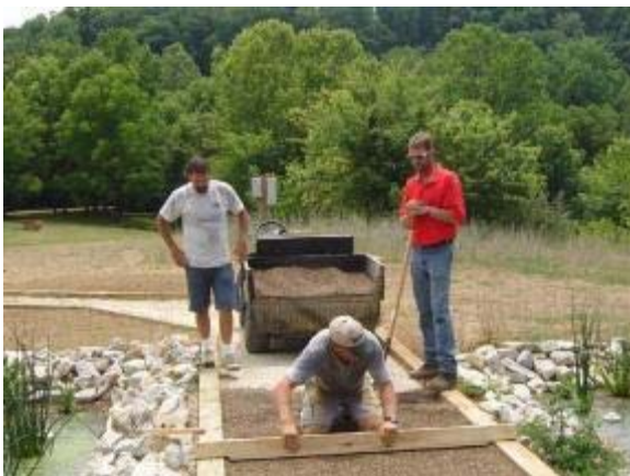
Photo 5 Klingstone top dress ¾ inch washed pea gravel is leveled. June 16, 2007.
