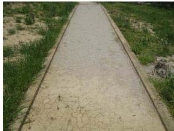
Photo 37 Soiltac Powder Mix-In softened surface would become firm again. May 6, 2008.
