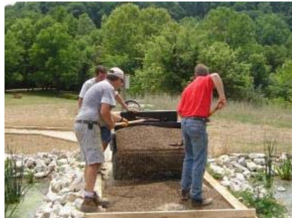
Photo 4 Klingstone top dress ¾ inch washed pea gravel is prepared. June 16, 2007.
