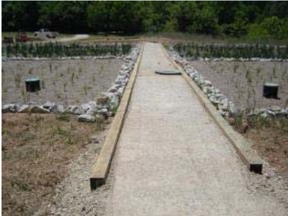
Photo 1 Klingstone base preparation of ¾ inch minus limestone and dust. June 13, 2007.
