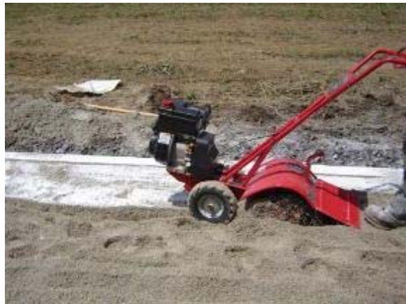
Photo 31 Soiltac Powder Mix-In has a penetration depth of 4 inches. June 27, 2007.
