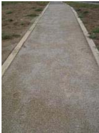
Photo 135 Quarter Inch Minus Limestone trail segment maintained itself in dry temperatures. October 19, 2007.
