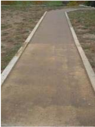
Photo 96 StaLok trail segment maintained itself through first round of testing. October 19, 2007.
