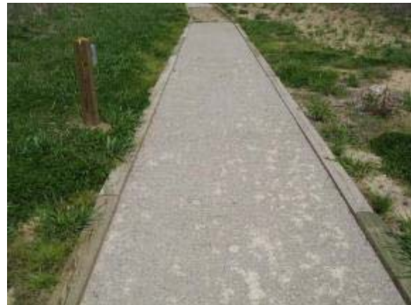
Photo 142 Three Quarter Inch Minus Base and Quarter Inch Minus Top Limestone trail segment firmed back up more quickly than the ¼ inch surface. May 6, 2008.
