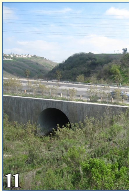
11 Environmental mitigation to address water pollution due to highway runoff or to reduce vehicle-caused wildlife mortality while maintaining habitat connectivity: Runoff pollution mitigation, soil erosion controls, detention and sediment basins, river cleanups, and wildlife crossings.
