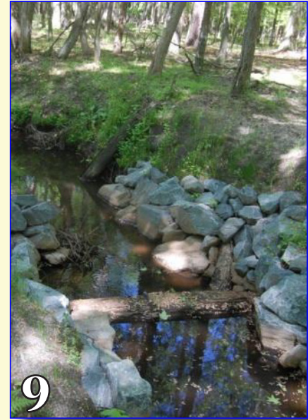
9 Stormwater Mitigation: Pollution prevention and abatement activities to address stormwater management; water pollution prevention related to highway construction or due to highway runoff.
