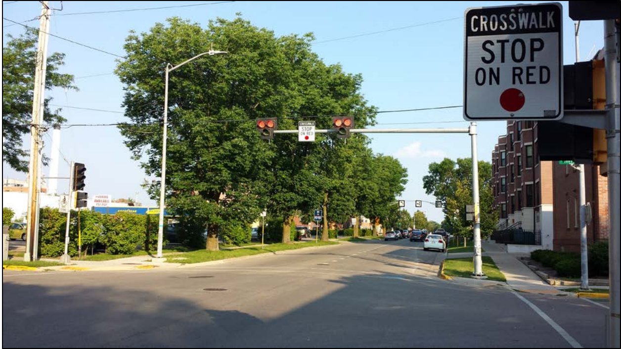
Figure 3.4: HAWK Signal Implemented in Field
