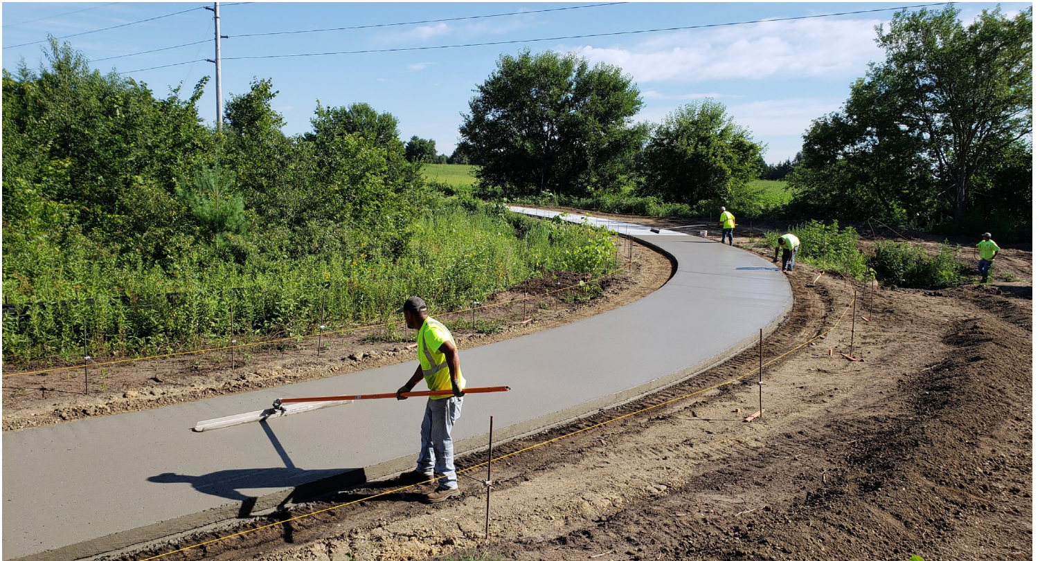
The Solon to Ely section of the Hoover Nature Trail under construction | Photo courtesy Johnson County Conservation Board
