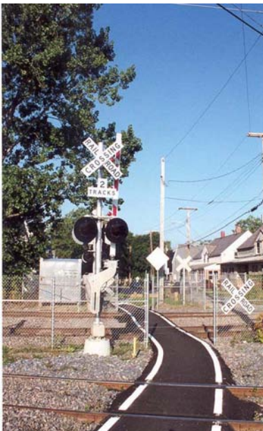
Along this trail in Burlington, Vermont, safety devices include cross bucks, flashing lights, a gate as well as a fence to encourage pedestrians to traverse the tracks at the designated crossing point.
