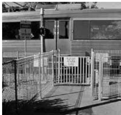
Gate closes automatically when a train approaches
