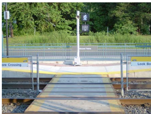
The audible device announces the approach of a train.
