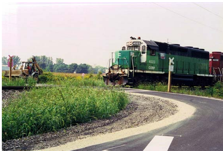
The Simon Kenton Trail in Ohio uses only cross bucks as safety devices. However, the trail curves intersecting the tracks at a right angle, slowing users and providing for an increased sight line. (Photo courtesy of Peggy Holland.)
