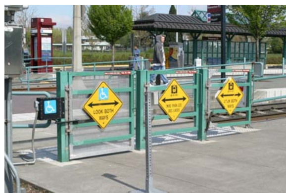
Disabled passengers and cyclists can use the push button control
