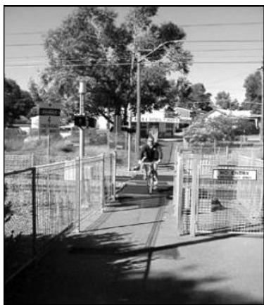
Perth Australia—City West Station. Automatic Swing Gate, which is normally open.
