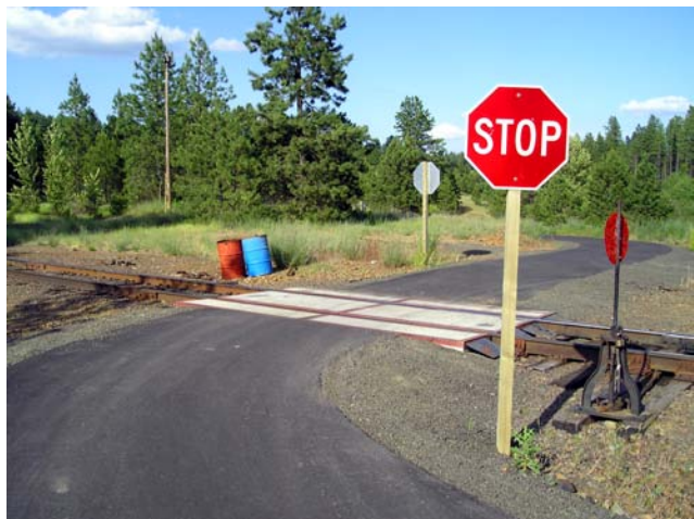
The 95 mile Trail of the Coeur d'Alene crosses the active St. Maries Railroad near Plummer. Safety devices are limited to railroad advance warning signs, stops signs, and a curve in the road to slow bicyclists. (Photo courtesy of Brian Momberg, RTC.)
