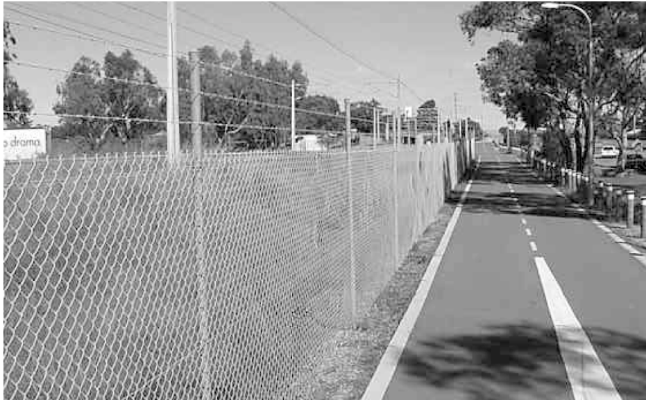
A section of RWT in Perth illustrates typical design and construction parameters, including 3 m (10 ft) wide asphalt path, set back from the adjacent rail line, and a 1.8 m (6 ft) chain link fence with three strands of barbed wire. Perth, Australia
