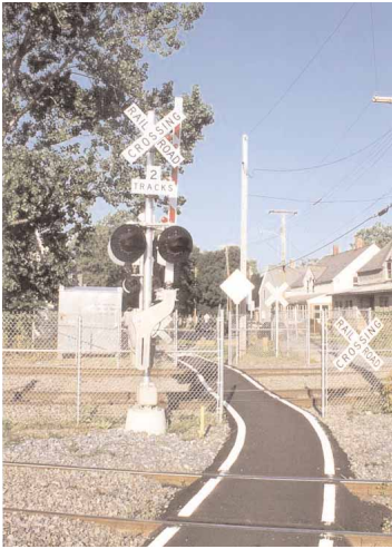
Dual track grade crossing. Burlington, VT
