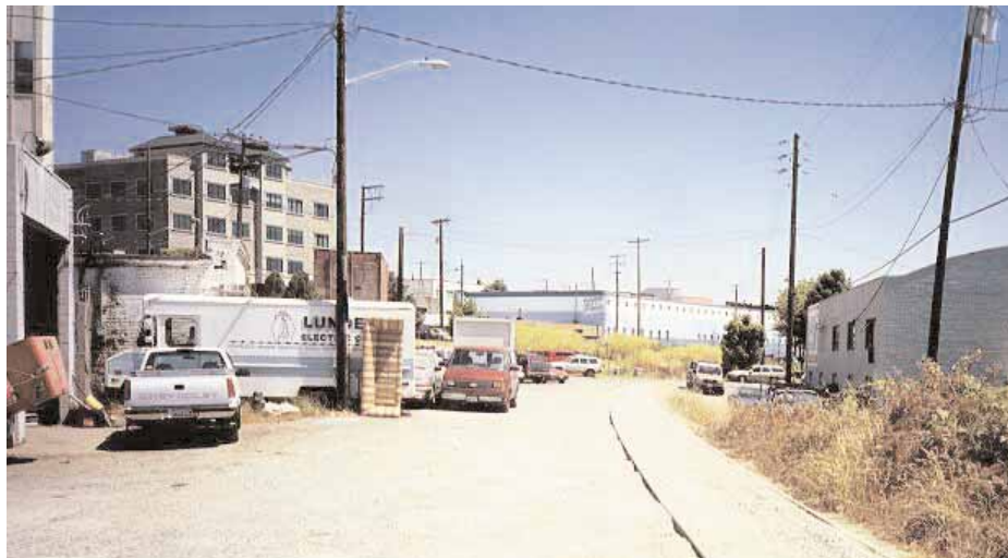
Planned future site of the Burke-Gilman Extension along the BTR tracks. Seattle, WA
