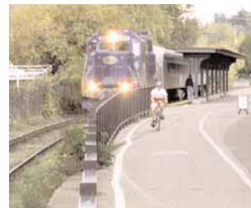
Burlington Waterfront Bikeway located along the Vermont Railway Company tracks. Burlington, VT
