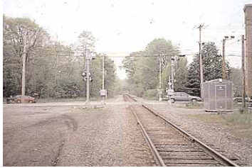
Location of the future Blackstone River Bikeway along the PWRR tracks. Albion, RI
