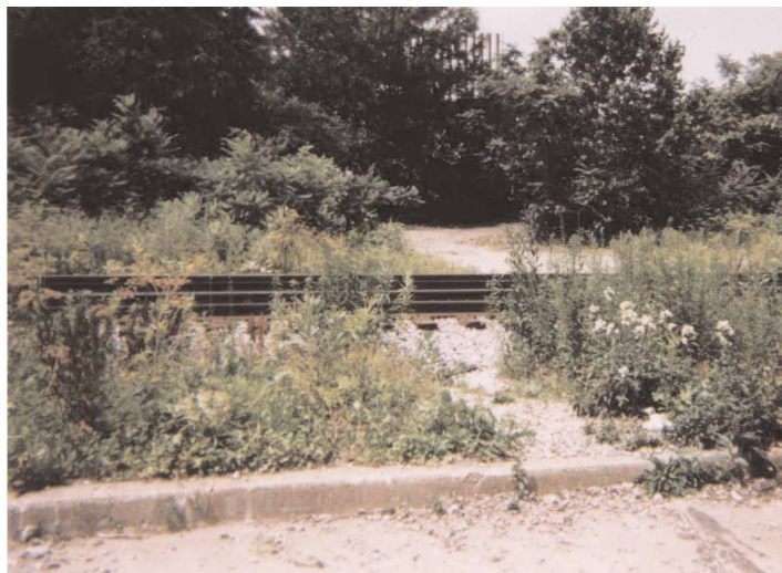
Current illegal crossing location over CSX tracks on Three Rivers Heritage Trail. Pittsburgh, PA
