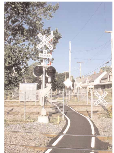
Dual track grade crossing. Burlington, VT
