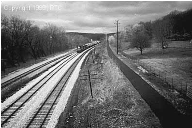
Copyright 1999, RTC Setback of 7.6 m (25 ft) or greater is often needed for higher speed train corridors. Stavich Trail, OH and PA
