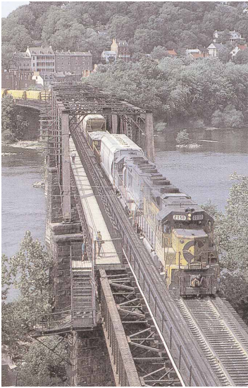
Harpers Ferry Bridge. Harpers Ferry, VA
