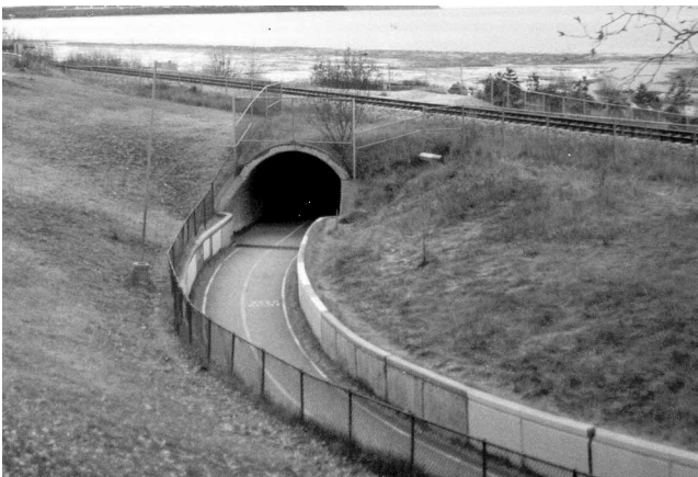
Undercrossing of Alaska Railroad Corporation tracks, Tony Knowles Coastal Trail. Anchorage, AK
