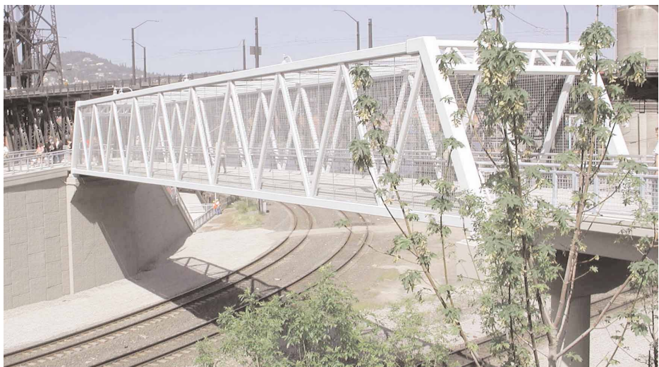
Bridge over Union Pacific tracks. Portland, OR
