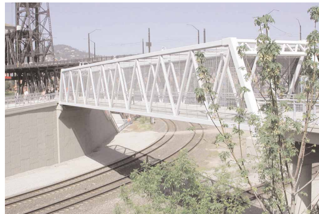
Overcrossing of Union Pacific tracks. Portland, OR
