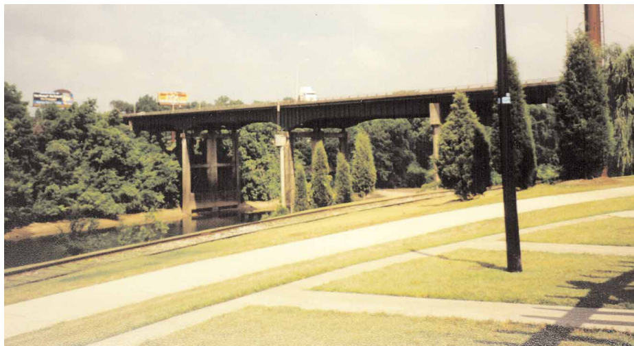
Columbus Riverwalk (Chattahoochee Trail) segment located along Norfolk Southern tracks. Columbus, GA
