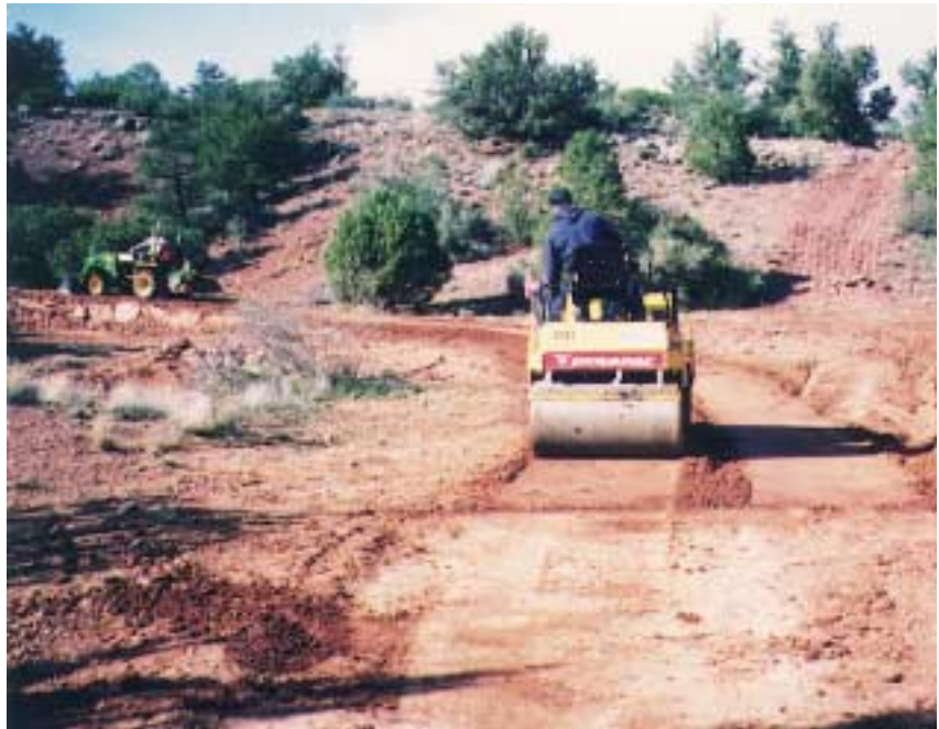
Figure 1. Equipment working on the Bell Rock Pathway on the Coconino NF.
