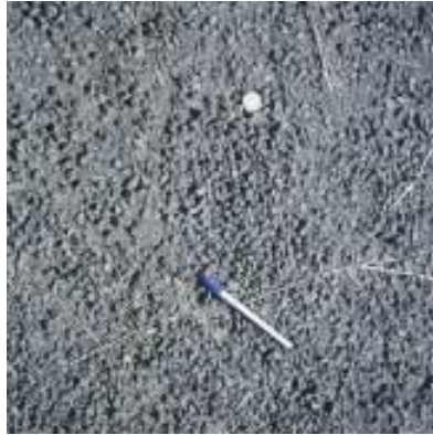
Figure 6. Macadam surface with blotter sand blown away.
