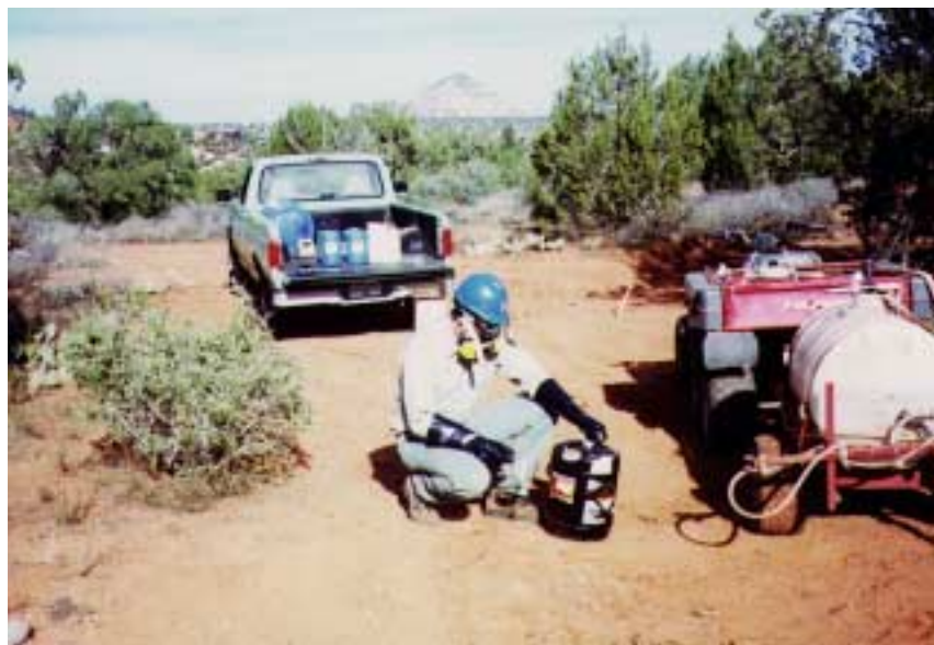
Figure 4. Bentonite with Roadbond EN-1 being applied to trail. Note that the worker is wearing the required PPE.
