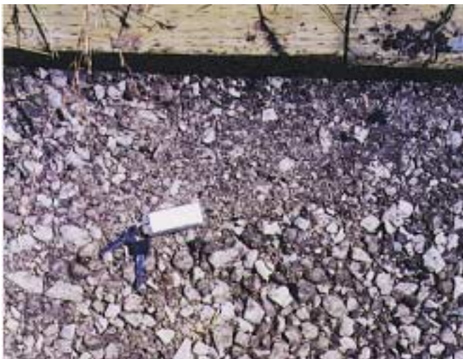
Figure 7. Coarse materials and loose surface rocks make it difficult to turn the wheels on a chair or walker.
