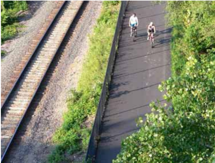
Trail built on a cut slope with fence along a rail in St. Paul, MN (Source: www.americantrails.org )
