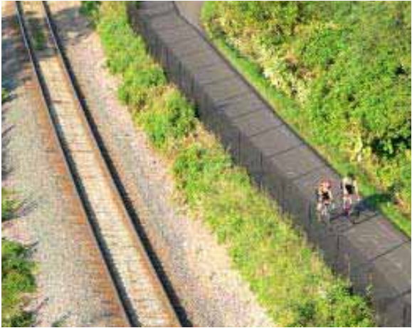
An existing rail-with-trail using vegetation and fencing for separation ( www.americantrails.org )
