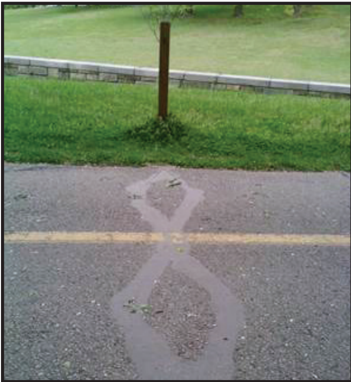
This permanent count station features a passive infrared counter housed in a wooden post and diamond-shaped inductive loops installed beneath an asphalt trail.
