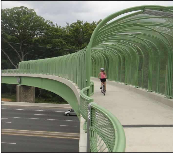
Pedestrian and Bicycle Facilities: Providing new or reconstructed sidewalks, walkways, curb ramps, bike lane striping, paved shoulders, bike parking, bus racks, off-road trails, bike and pedestrian bridges and underpasses
