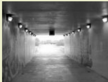
The I-90 tunnel in Washington utilizes two security cameras, one of which is visible on the ceiling of the tunnel. Credit: Washington State Department of Transportation.
