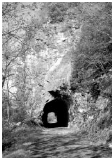
The Austinville Tunnel along the New River State Trail in Virginia is an example of a “mined” tunnel. Credit: Virginia State Parks.
