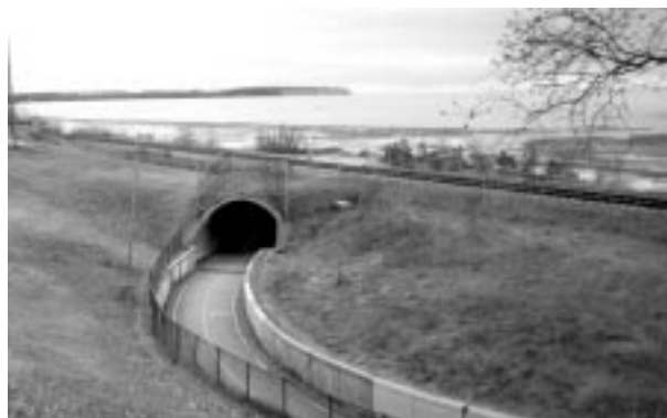
This is an example of a “cut and cover” tunnel. Tony Knowles Coastal Bike Trail, 10 Anchorage, Alaska. Opened 1987. Credit: Jack Mosby.
