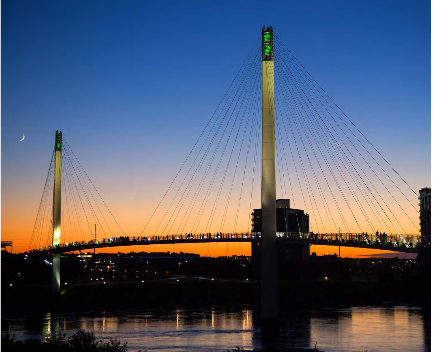
Bob Kerrey Pedestrian Bridge connecting Iowa and Nebraska | Photo by Matthew Nissen
