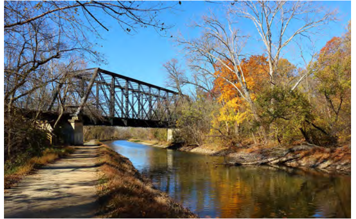
C&O Canal National Historical Park traveling under the Capital Crescent Trail | Photo by Alice Crain
