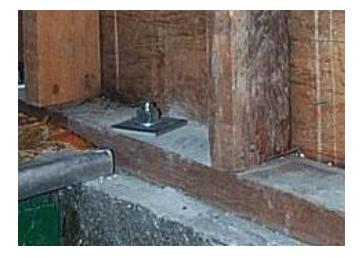
(Below) Foundation anchors help keep the building tethered to its foundation during a seismic event. Ideally they are coupled with a continuous perimeter foundation.
