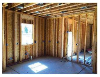
(Above) Plywood shear walls reinforce the first floor of a wood frame building. They help prevent lateral shifts and transfer seismic loads. They can be made from plywood, masonry, or concrete.
