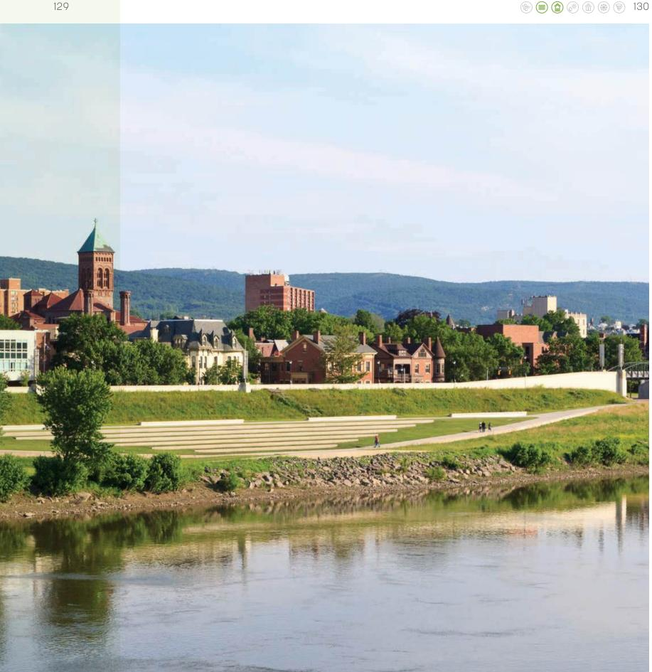
have the advantage of a smaller footprint and more structural stability. Since they are made with stone and concrete, flood walls can often be incorporated into the architectural design of a site. The main disadvantage to flood walls is that they tend to cost more than embankments.
