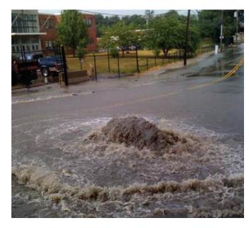
Intense rains can cause the sanitary and storm sewers to combine and overflow together.
