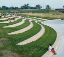
(Bottom Left and Right) Photos of site and integration of seating and public-use elements into design of levee. Source: Sasaki
