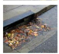
(Left) Gutter clogged with debris, causing local flooding. Source:
