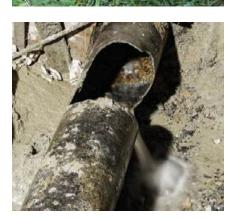
(Left) Old pipes corrode and break, causing system disruptions and local flooding.
