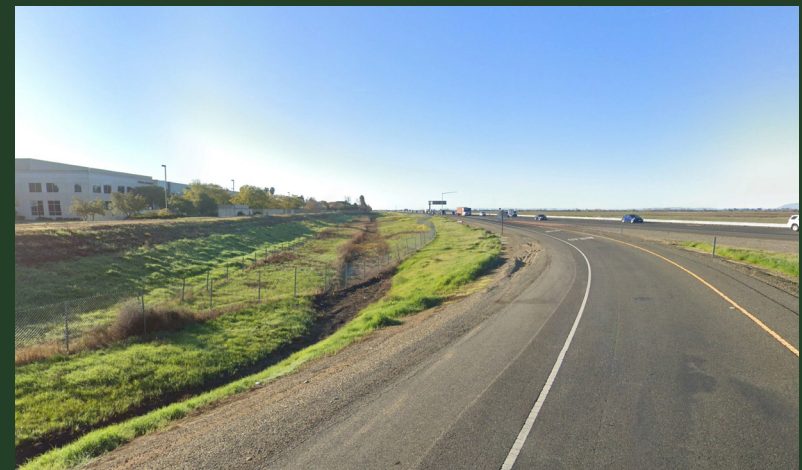
View of I-5 and the adjacent levee, looking south. Source: Google StreetView.
