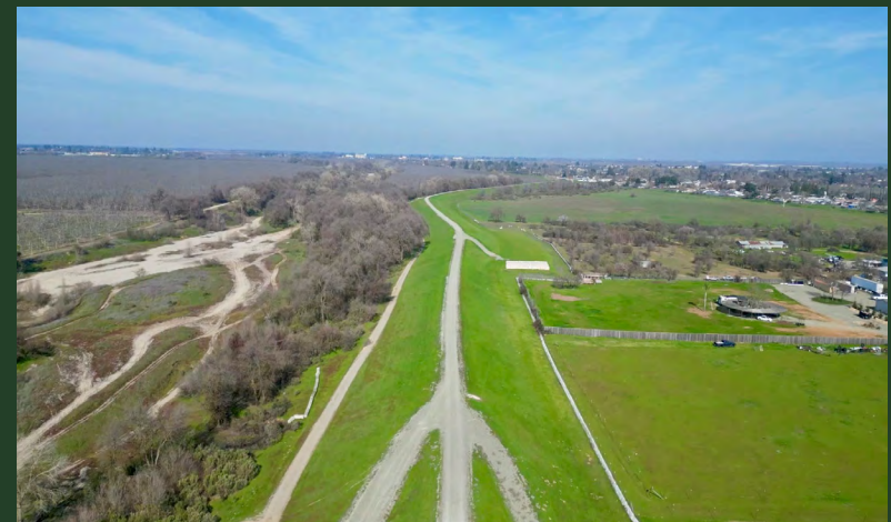
Existing Levee Path looking north (Source: Yuba County)
