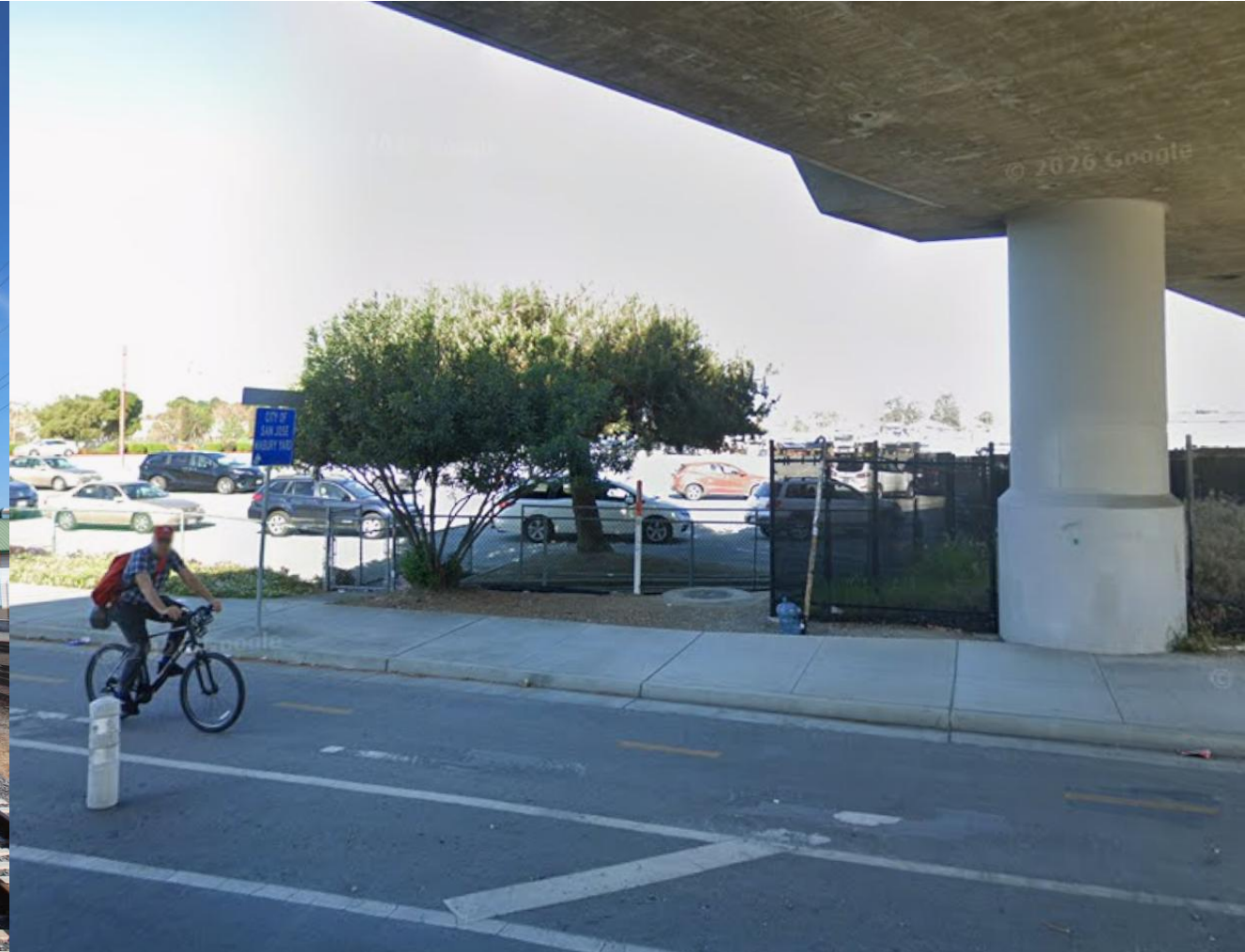
On-street segment + highway undercrossing
